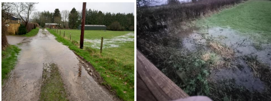
Pond created by storm water on north side Hopyard Cottage
