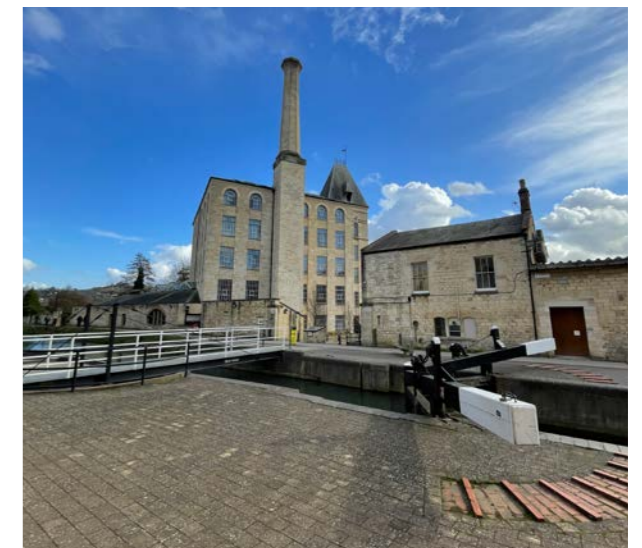
▲ Restoration of the Stroudwater Navigation at Ebley Wharf, Stroud.
