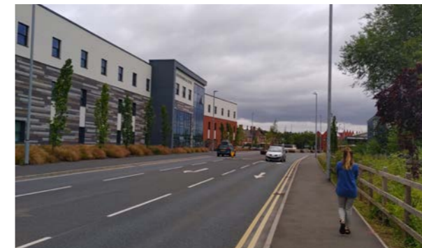
▲ The existing Link Road is unsafe and unfriendly for walking and cycling.
