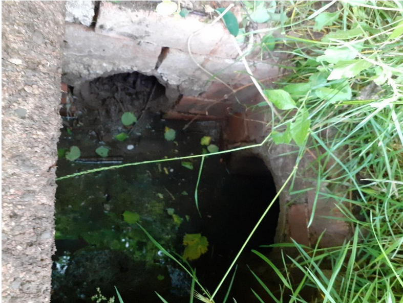
Existing highway drainage catchpit showing pipe below the highway, noting that the inlet is not visible
