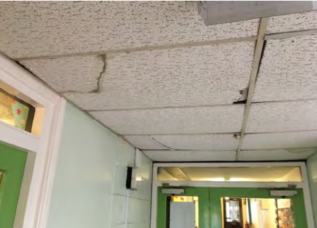
Ceiling tiles- require replacement
