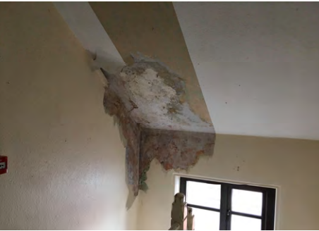
Severe water damage above staircase
