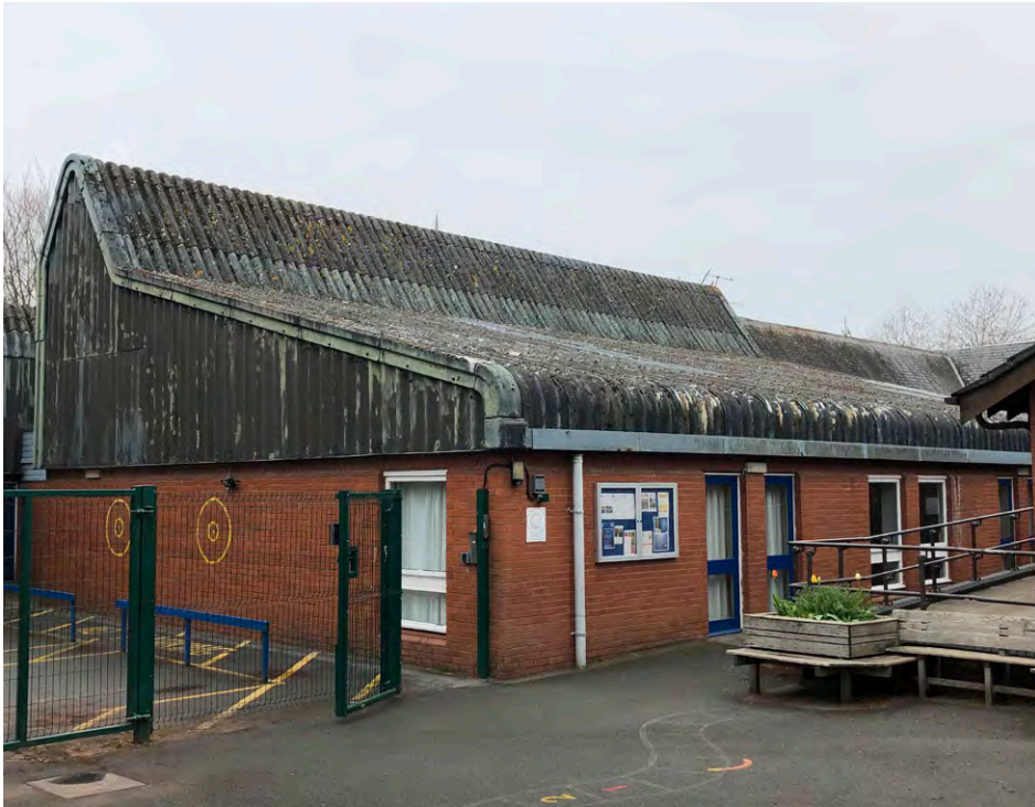
Asbestos cement sheet roof to hall and classrooms to the front of the site
