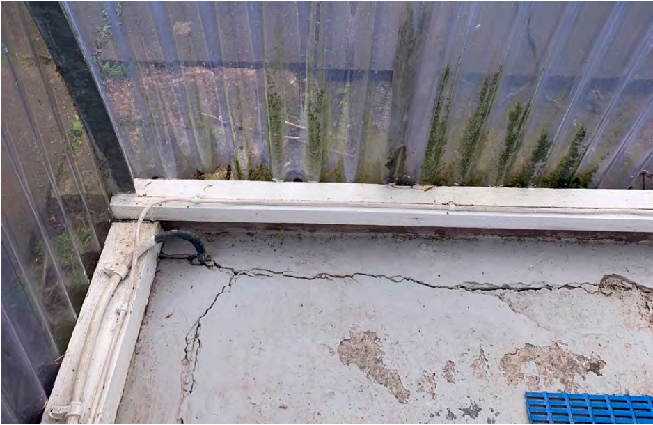
Cracked concrete floor to the swimming pool, with algae growth on the polytunnel roof.
