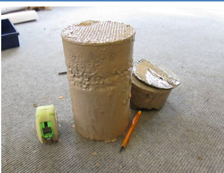
Representative photograph depicting a concrete core from the coring of WS7 within the school building. The concrete was found to be 0.18 metres thick within WS6, 0.32 metres in WS7 and 0.30 metres thick in WS8.
