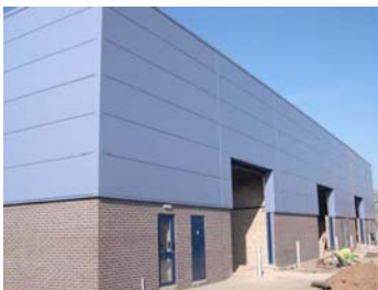
Twyford Road units nearing completion
