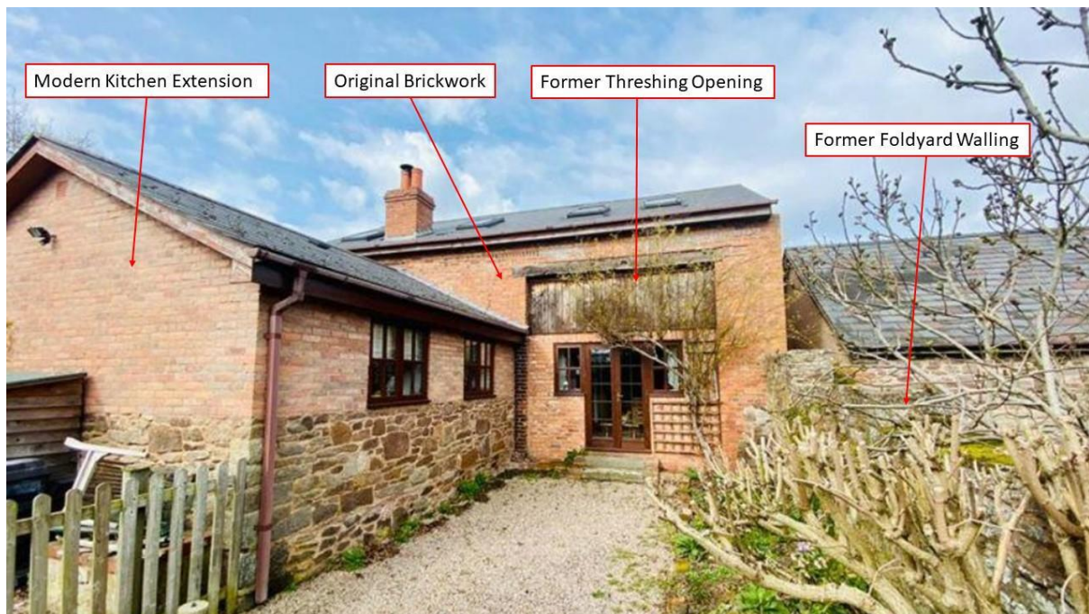
Original Brickwork & Vertical Brick Pier
